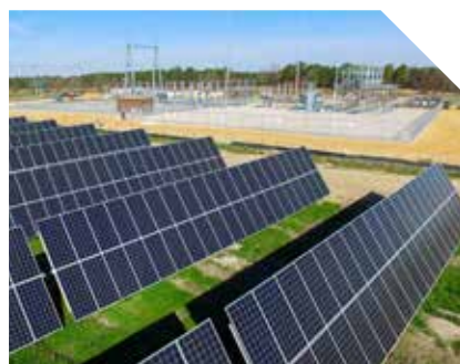
NC-31 Block 16 and substation - March 2017
