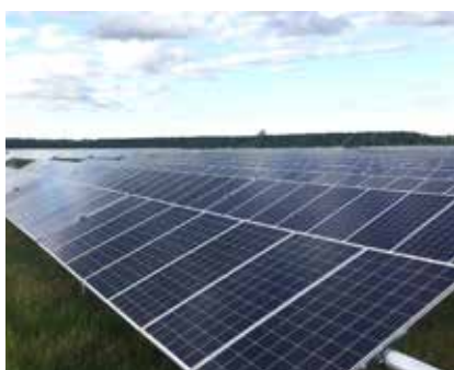
NC-47 ground view - May 2017
