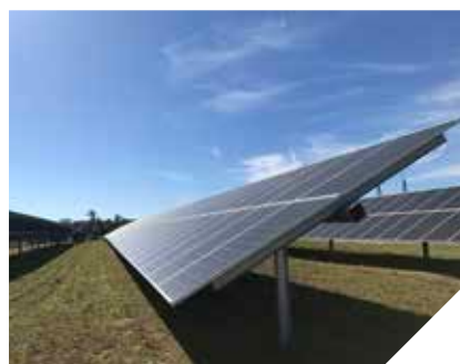
NC-31 ground view - October 2017
