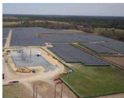
NC-31 array and substation - aerial view - March 2017
