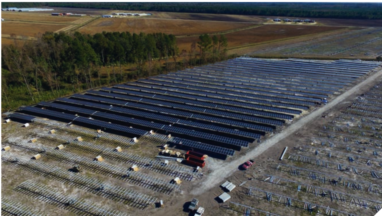
NC-31: Installation of racking and mounting of solar panels is in progress (photo taken November 2016)
