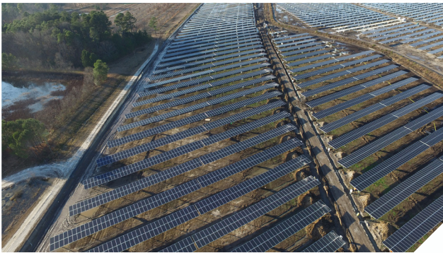
NC-31: View of Block 12 of the site
