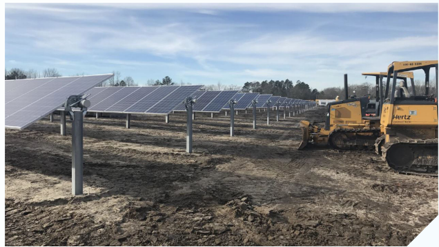
NC-47: Panel installation
