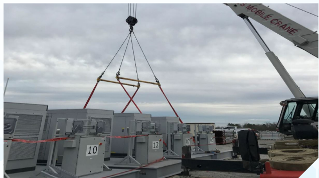
NC-47: Inverter being loaded for install
