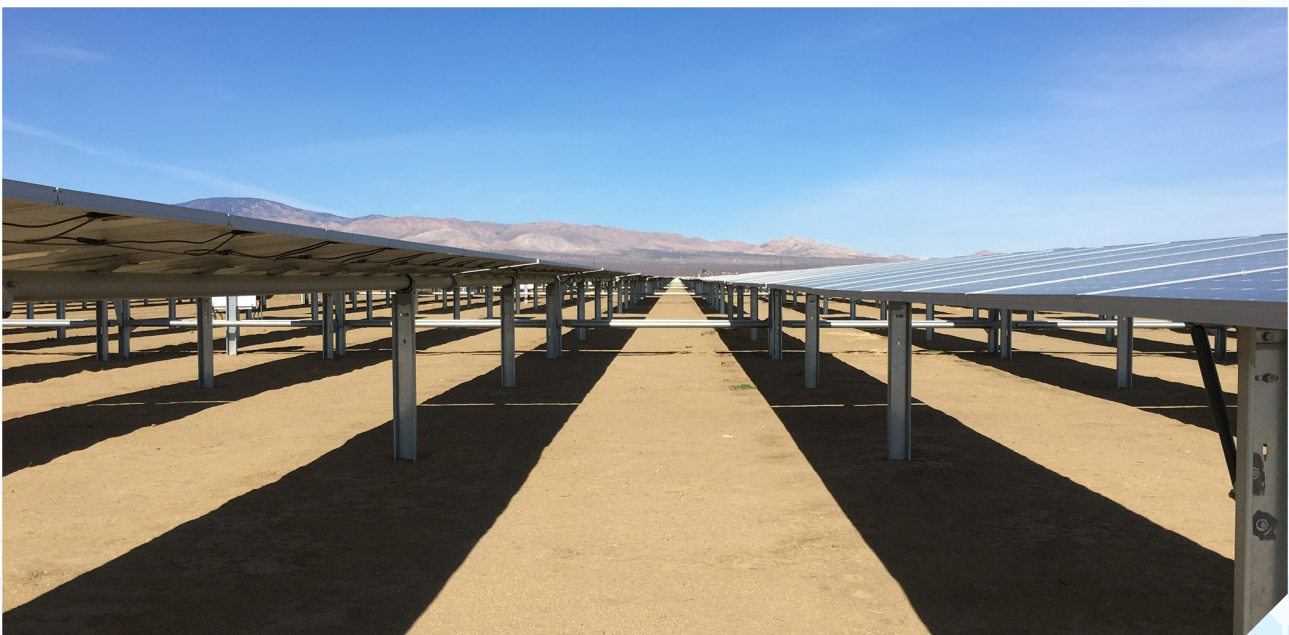
Stanford SGS: Solar panels tilting to follow the sun
