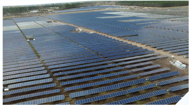
NC-47: Block 11 during construction
