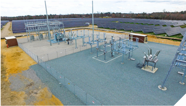
NC-31: Duke substation
