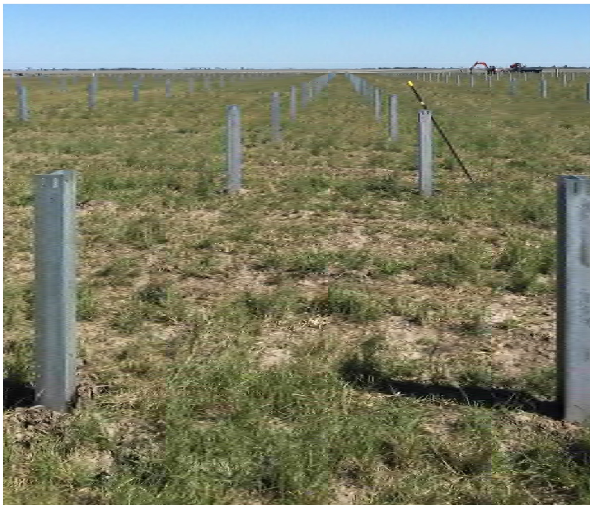
a) Driven piles (these may also be screwed into the ground).
