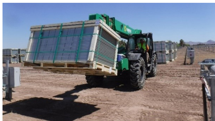
Initial delivery of modules to the MS2 construction site.
